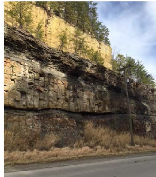
Figure 9: Rock Cut on Trus Joist Lane Near KY 15
