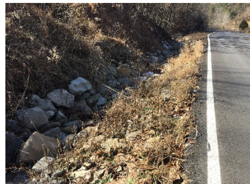
Figure 2: Terminal Road; Edge of Pavement
